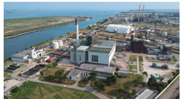
Marghera power plant.
