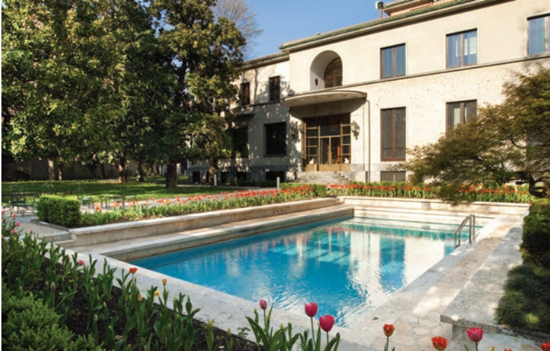
Villa Necchi Campiglio, the 1930s Art Deco icon in Milan. A FAI treasure, which is also supported and protected by Edison through energy efficiency measures.
