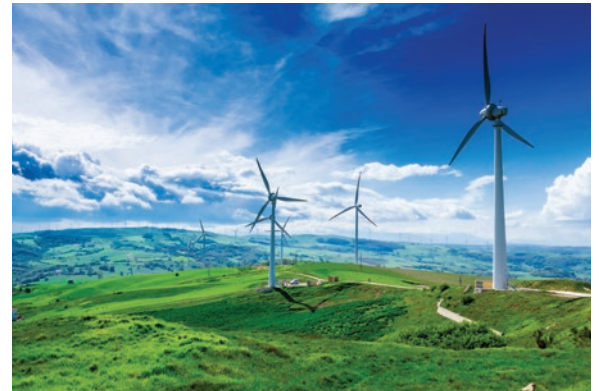
Renewable energy. Edison's wind farm in Foiano di Val Fortore in Campania.
